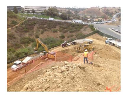
**Photo 2:** Haul trucks being loaded with soils for export offsite via use of an excavator. A paleontologist can be seen in this photo overseeing construction activities in accordance with APM-CUL-1.
