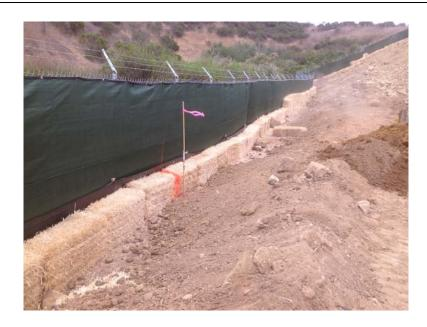
**Photo 4:** BMP's consisting of hay bales and silt fence installed along the downslope perimeter of the project site in accordance with the Stormwater Pollution Prevention Plan (SWPPP) and MM-HYD-1.
