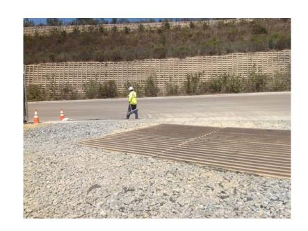
**Photo 3:** A rattle plate and rock apron being maintained at the project entrance to minimize tracout. A construction crewmember can be seen in this photo sweeping Mira Sorrento Place to remove trac-out.
